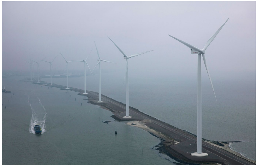
Delfzijl wind farm in the Netherlands (63 MW for Google)
