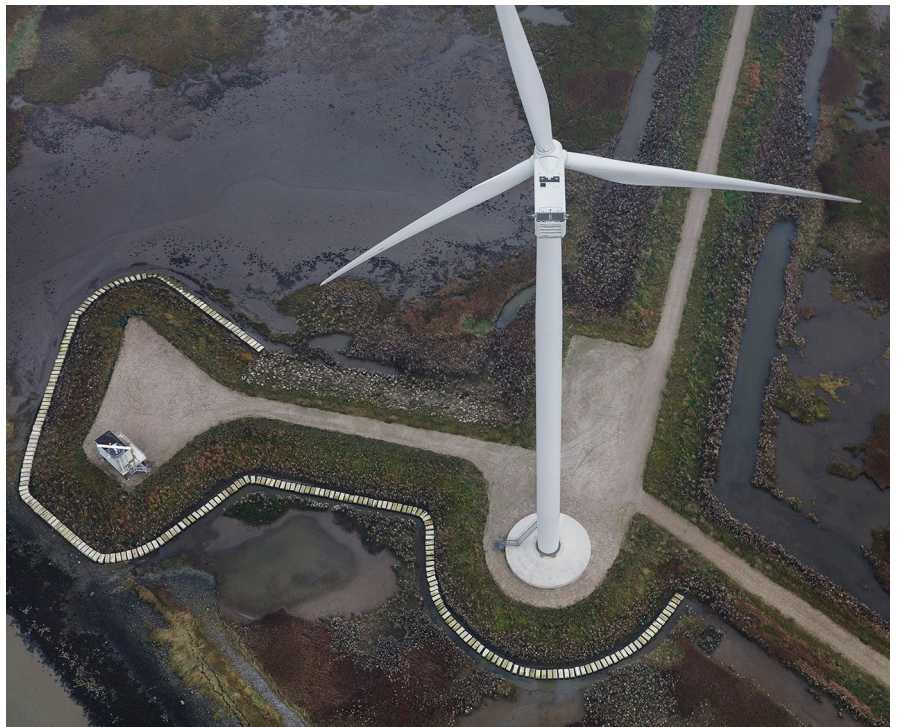
Delfzijl wind farm in the Netherlands (63 MW for Google)
