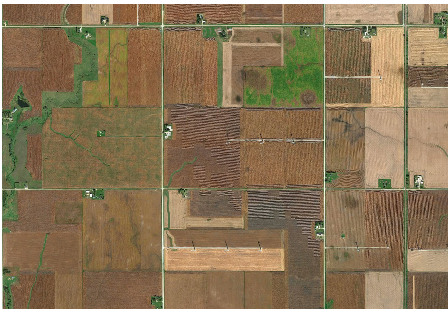
Story County II wind farm in Iowa (114 MW for Google). Imagery and map data: Google
